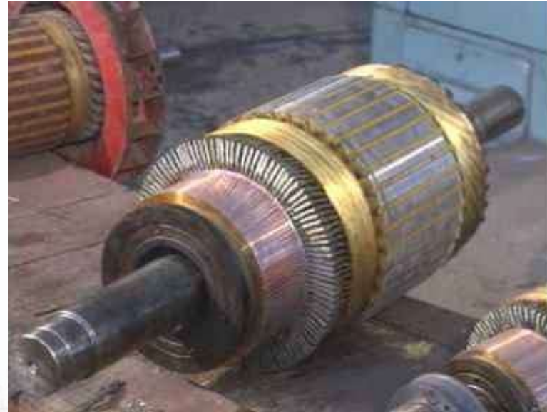
Rotor oil and dust cleaning
