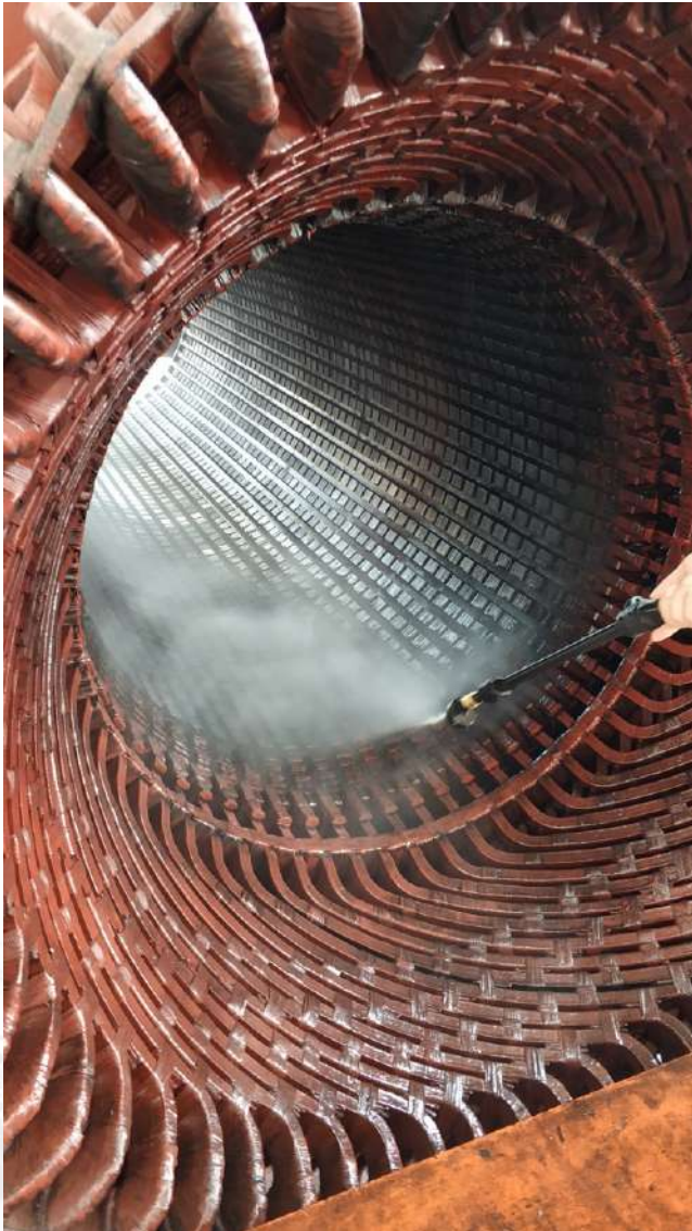
Dust cleaning of motor stator
